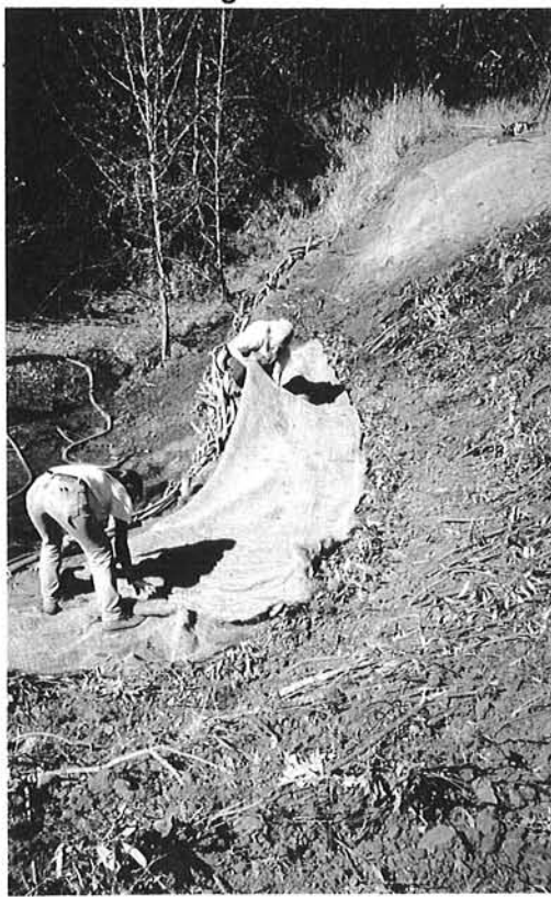
Installing the coir cloth
